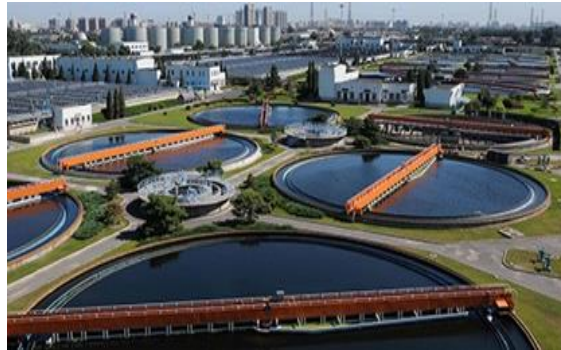
Waste Water Treatment Plant
