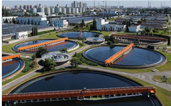
Waste Water Treatment Plant
